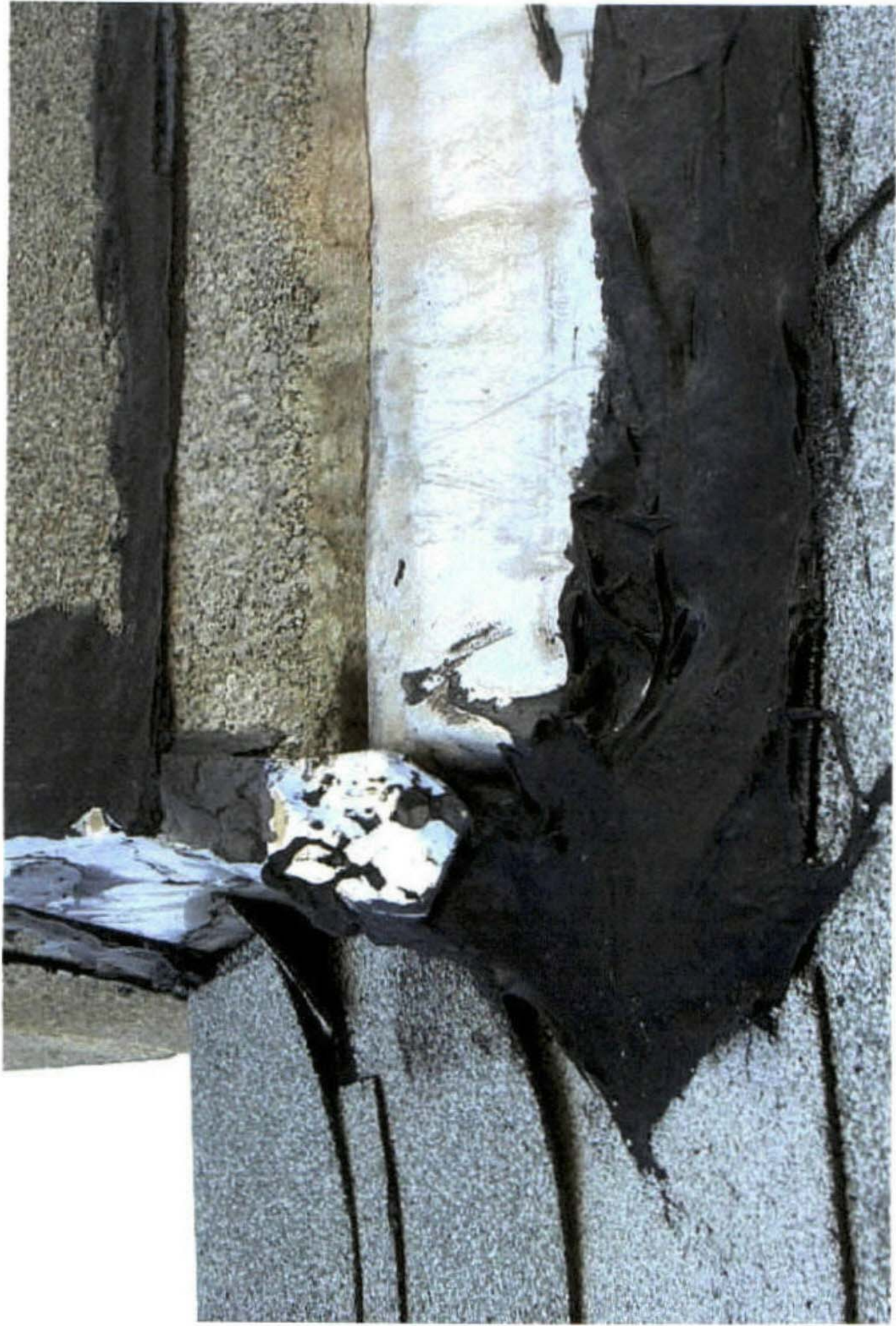
Shows use of gobs of tar and poor placement of one shingle. Note the tar is on top of the shingles (Photo by Professional Home Inspection Services)
