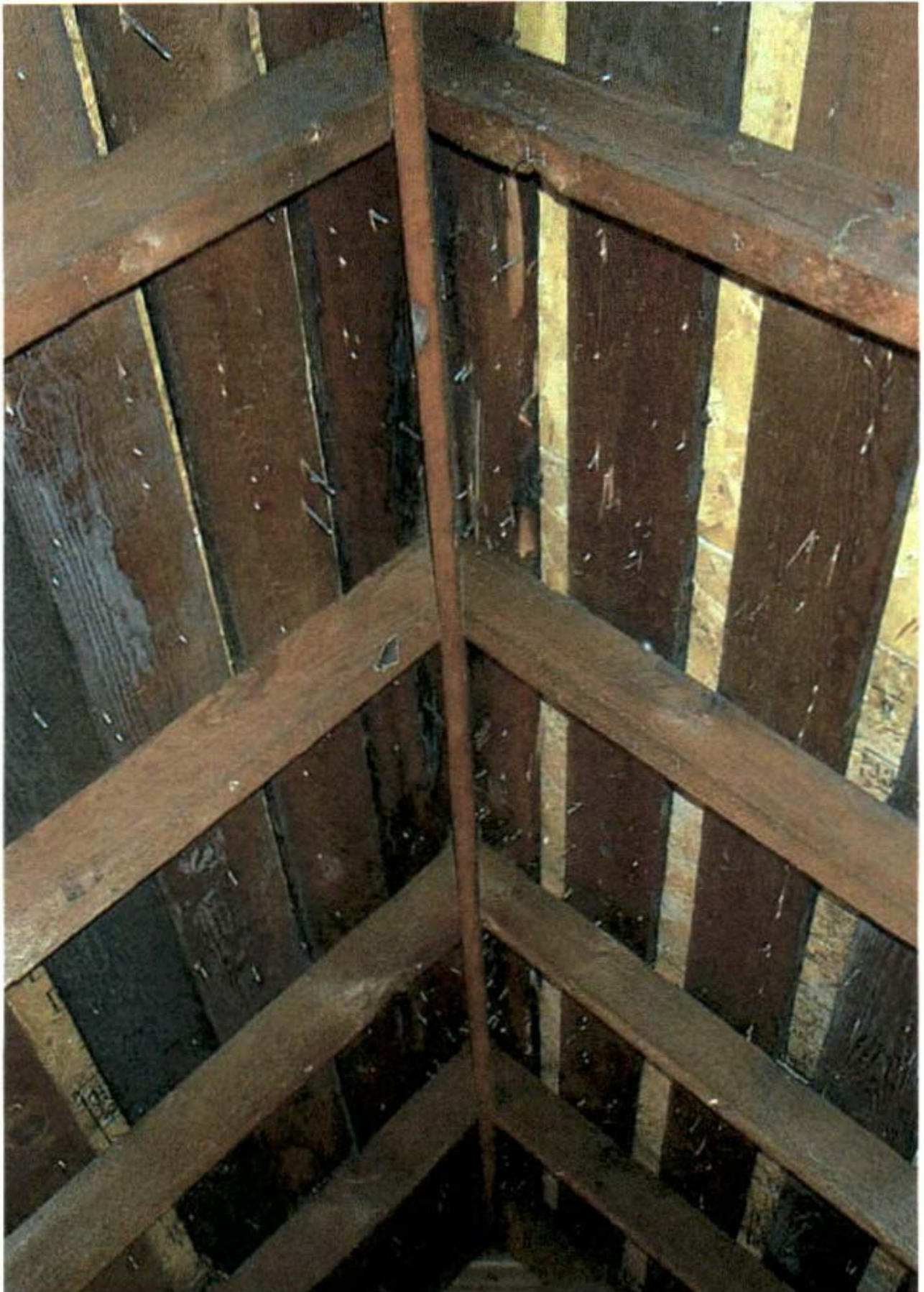
Attic framing was not cut through at any of the four peaks to allow warm air to flow out. Ventilation system purchased by homeowner is effectively non-existent. (Photo by Professional Home Inspection Services)
