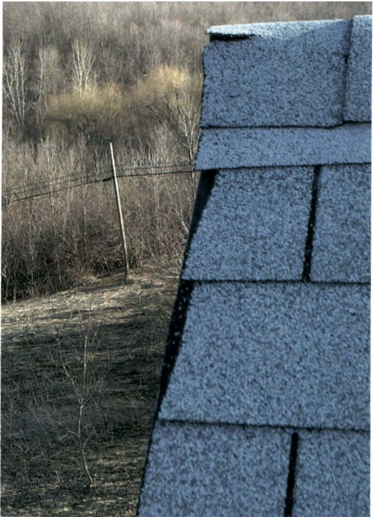
Jagged cuts on edge of roof; and a split ridge-cap right at the top of the peak (Photo by Professional Home Inspection Services)
