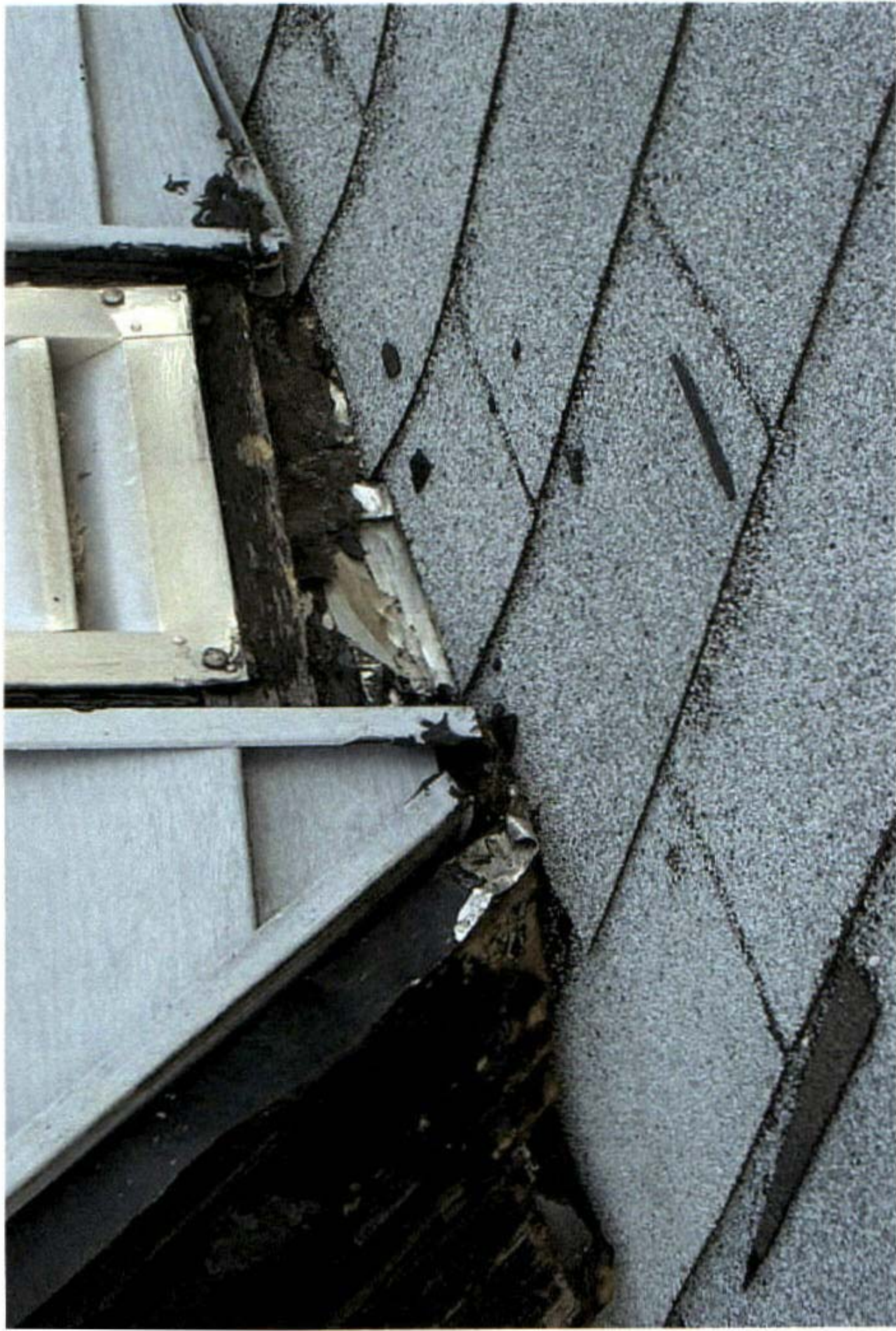
More debris and the flashing was not replaced as required by NYS code (Photo by Professional Home Inspection Services)
