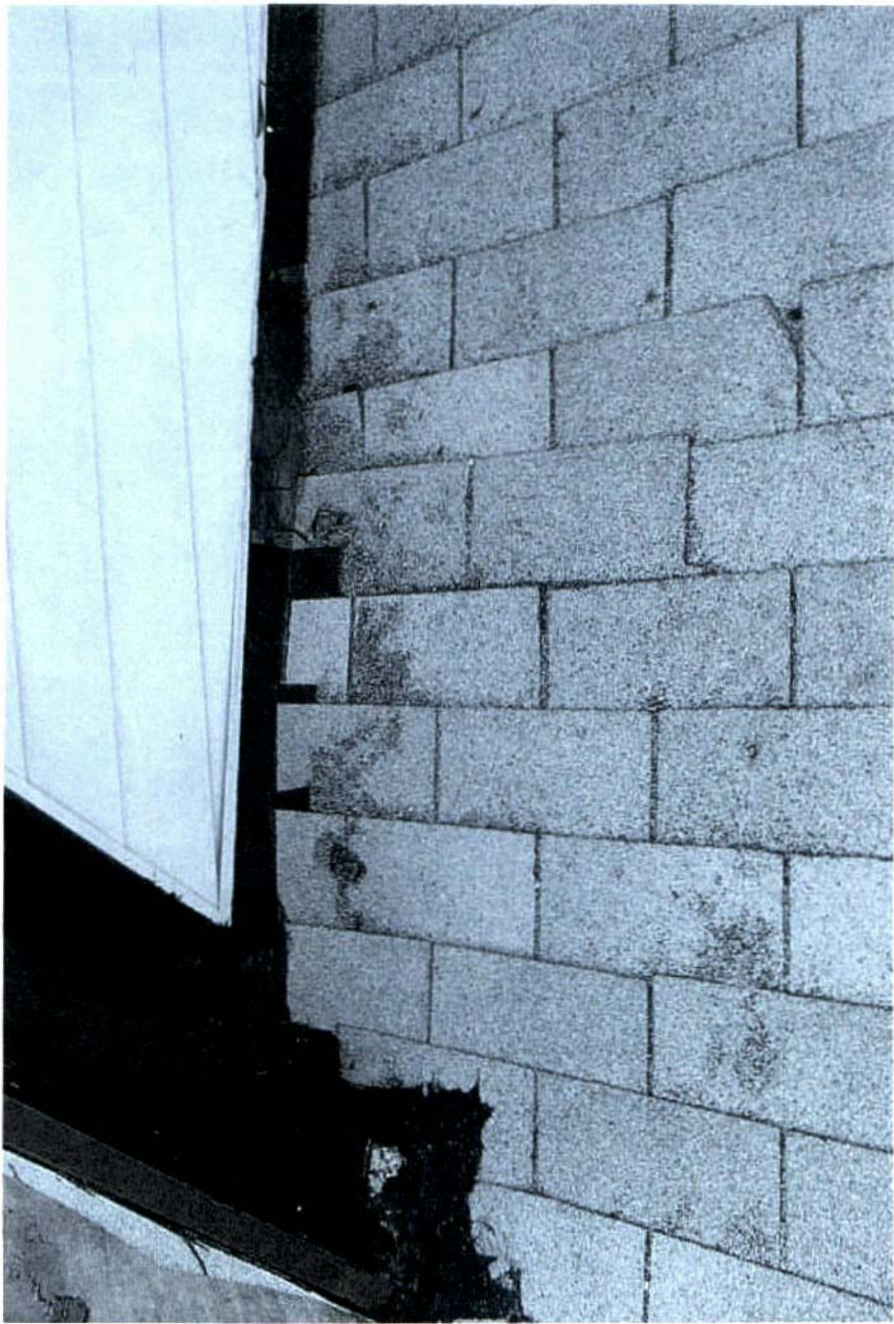
Sloppy work, use of tar instead of required new flashing, poor line up of shingles, and another gouged shingle (Photo by Professional Home Inspection Services)
