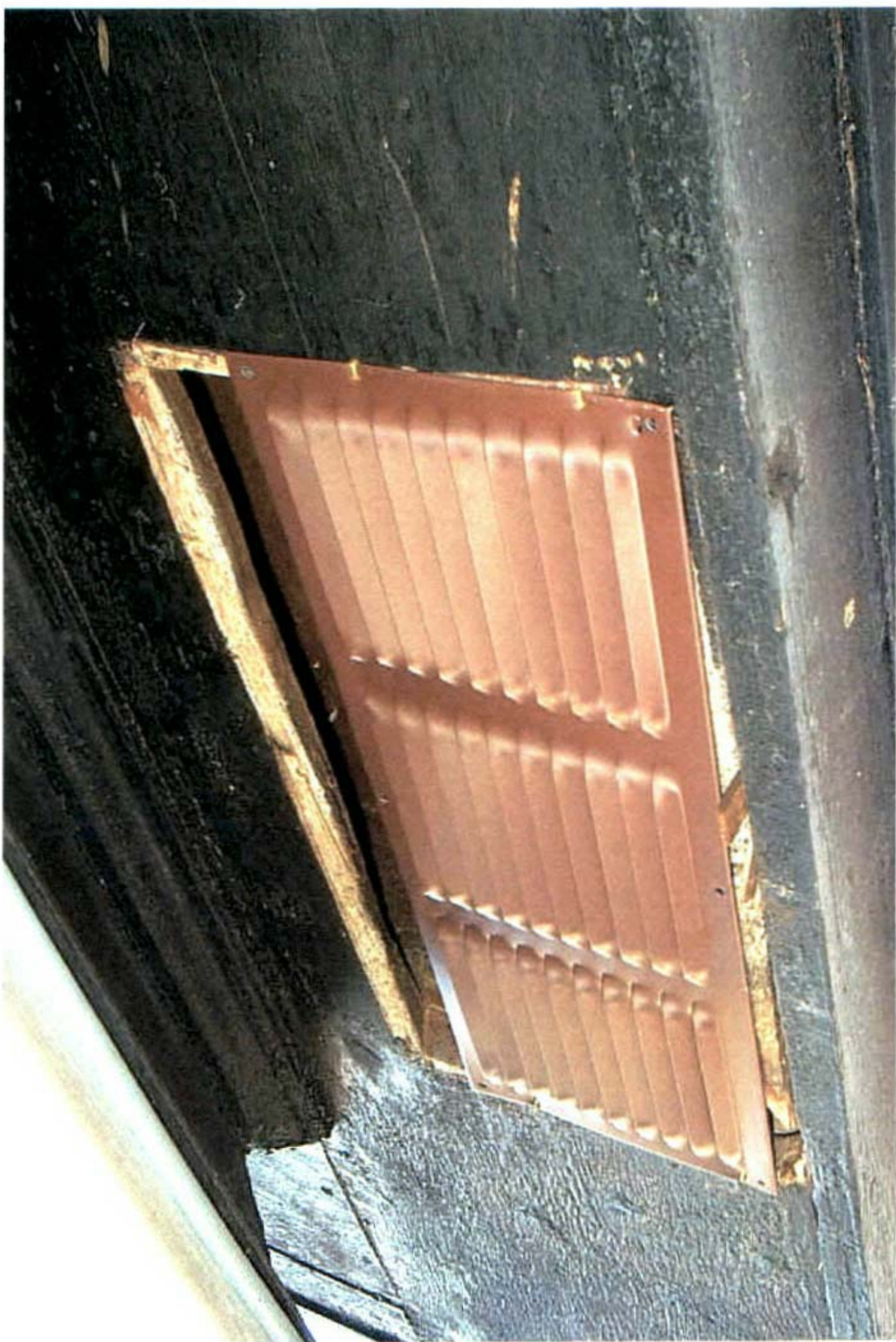
This shows how the crew installed a vent cover too small for the pre-existing hole. (Photo by Professional Home Inspection Services)
