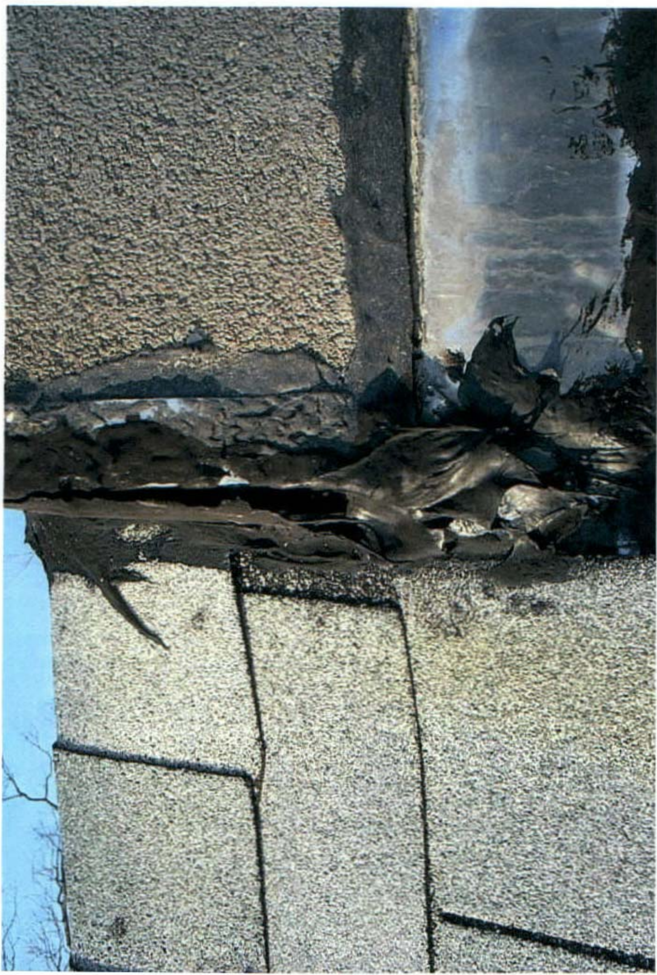
The crew used gobs of tar instead of required new flashing Notice the split in the old flashing – where the tar is leaking out. (Photo by Professional Home Inspection Services)
