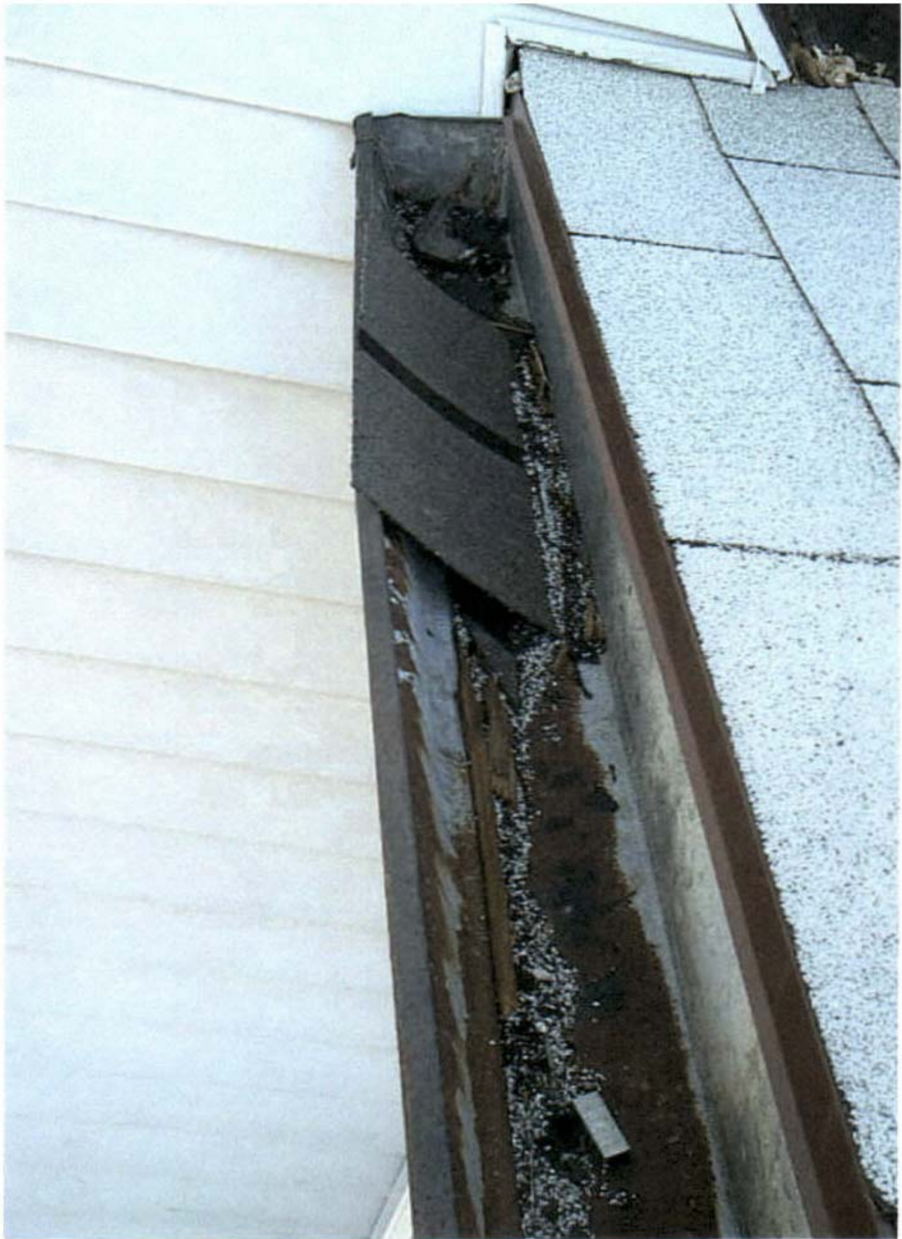
Debris that the crew left in one of the gutters. Shows that the roof is flush to the wall – no overhang into the gutters as dictated in the Manufacturer's specifications. Water will leak into the wall behind the siding. (Photo by Professional Home Inspection Services)
